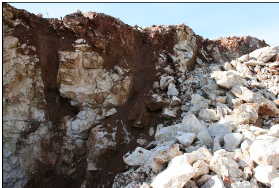
Figure 2: Limestone unit with crevices formed and filled with clay and silt
