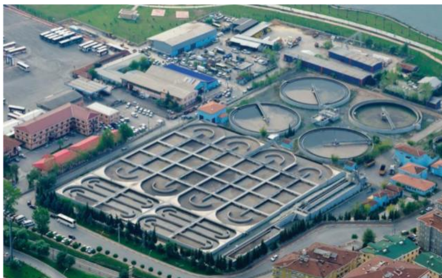
Figure 1: Plajyolu wastewater treatment plant
